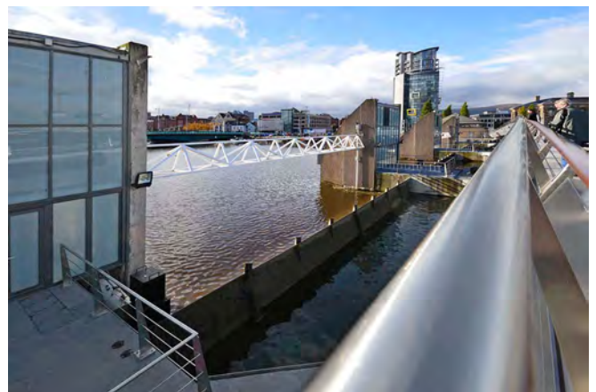
The view from the footbridge – the weir gates lifted and Pier House no.4 is nearest. The lattice girder between Pier Houses is a safety feature - when the weir is impounding water and cannot be crossed, the lattice girder is lowered via an electric winch system. The girders were an add-on to the weir’s original design but haven’t worked well and may be removed in the future
